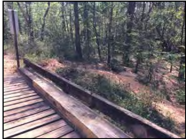
Figure 3-5C. Dorcas Road at Pond Creek Bridge with significant sedimentation next to the bridge.
