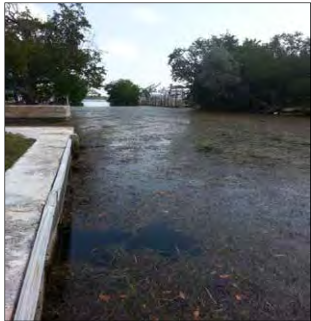
Figure 23-1B. Poorly flushed canal with excessive decaying vegetation.
